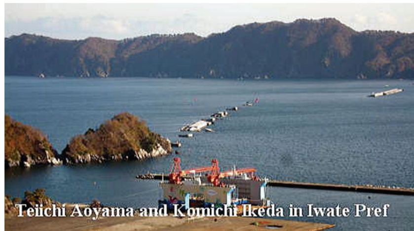
Fig.5. The breakwater at the entrance of Kamaishi bay destroyed by the tsunami (Construction cost: 120 billion yen)
