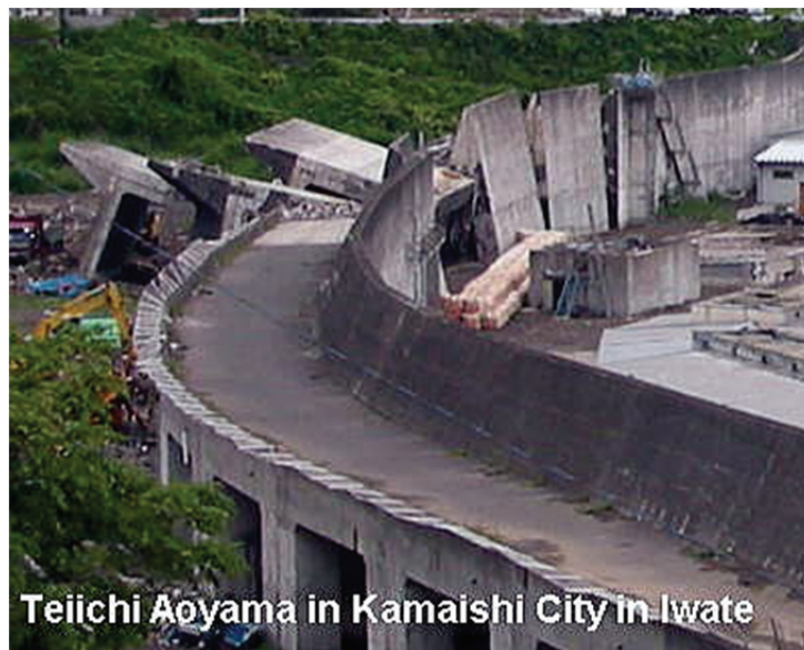
Fig.6. The tide embankment at Kojirahama fishing port in Touni Town, Kamaishi city, destroyed by the tsunami
